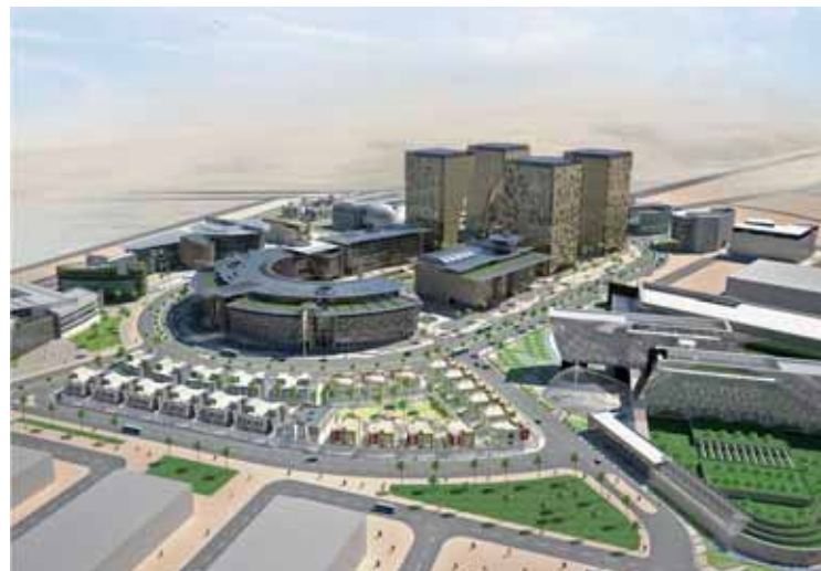
Riyadh. Der Information Technology and Communication Complex.
